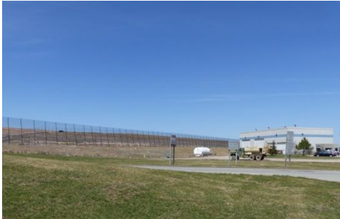
Fencing Along Residential Development
